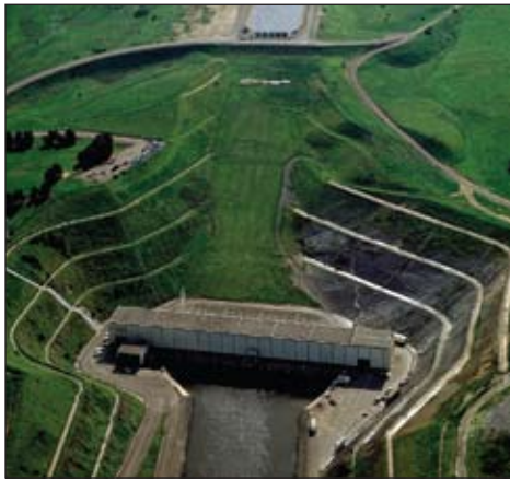
The Harvey O. Banks Pumping Plant in the south Delta is the starting point of the California Aqueduct, the world's largest water conveyance system, which delivers water to the Bay Area, the San Joaquin Valley, and Southern California.
